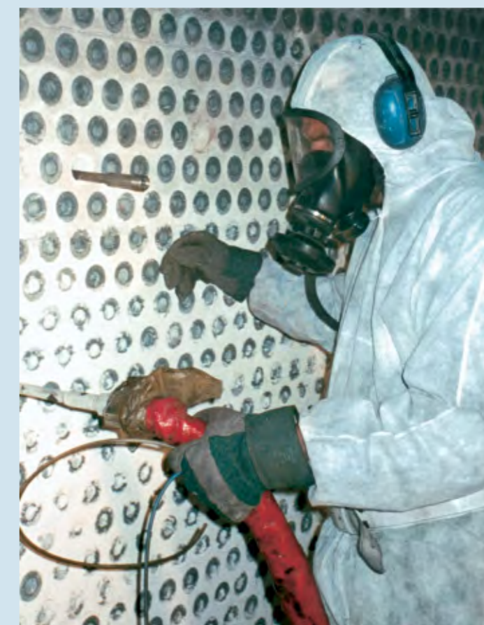
In some cases, gas masks are highly recommended – e.g. when cleaning heat exchangers and wherever harmful materials are blasted loose.
