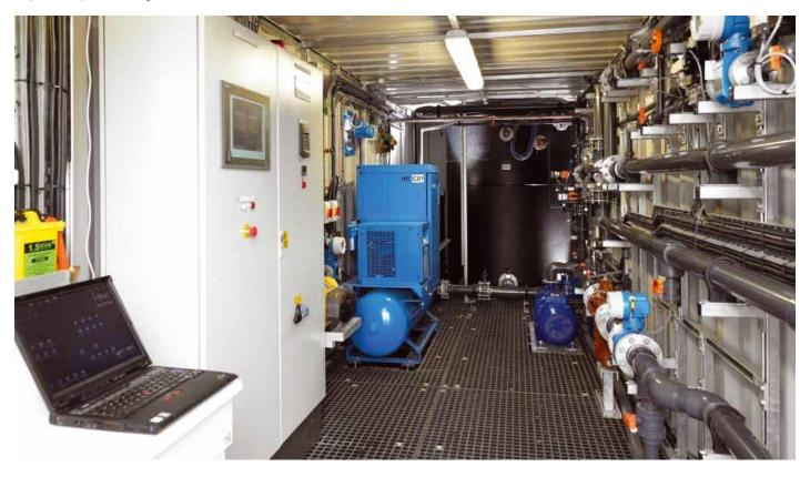
The evaluation is translated into the design of a containerised AXENIS™ solution which just requires a concrete pad on the customer's site near to the bioreactor and pipework interconnection, the footprint of which is much less than the space occupied by the conventional clarifiers.
